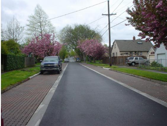
Figure 2: Permeable paving is an infiltration BMP. It is installed here in the parking lanes on a street.
